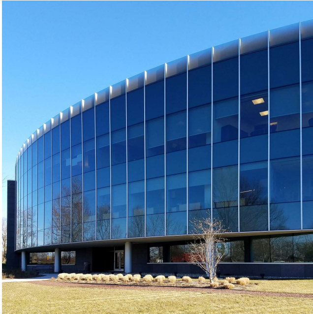
Photo: SCHWING Technologies North America Inc. office in Princeton New Jersey
