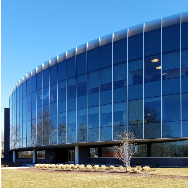
Foto: Büro SCHWING Technologies North America Inc. in Princeton New Jersey
